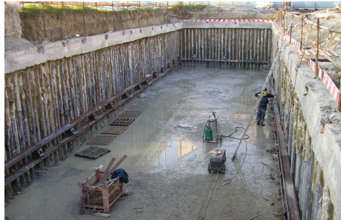
Embedded Retaining Walls
