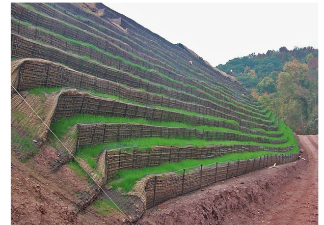
Reinforced Soil Slopes
