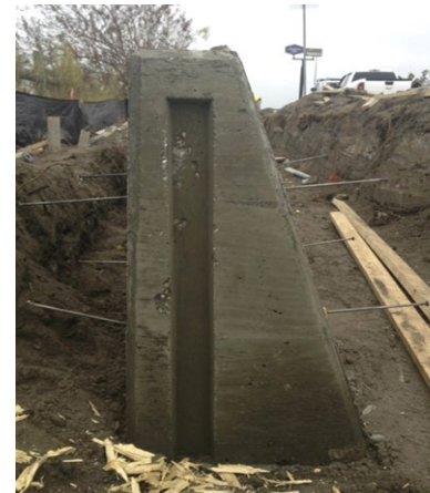
Gravity Retaining Wall
